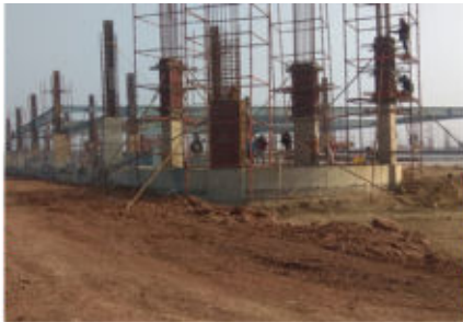
Column Casting (January 2023)
