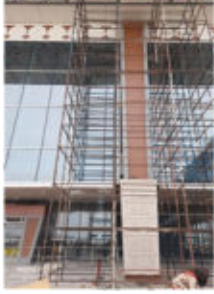
Column Cladding (January 2024)
