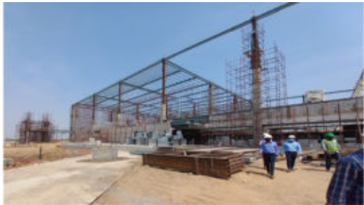
Super Structure (April 2023)
